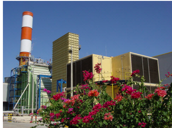
Thermoelectric Plant "Las Flores"
