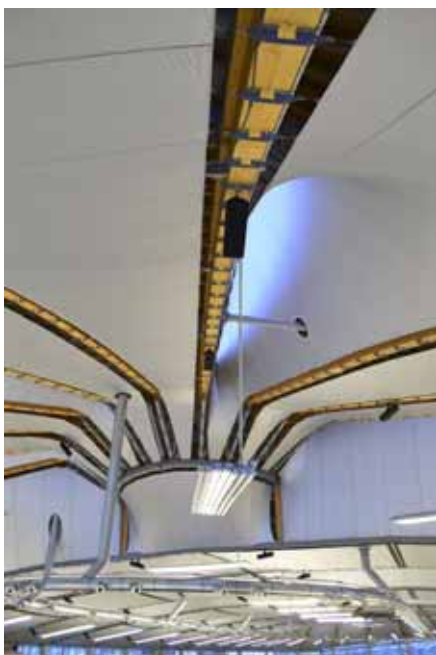
A total of eighty-nine Electro-Voice Sx600 loudspeakers provide sound reinforcement in the new 6,000-seater arena
