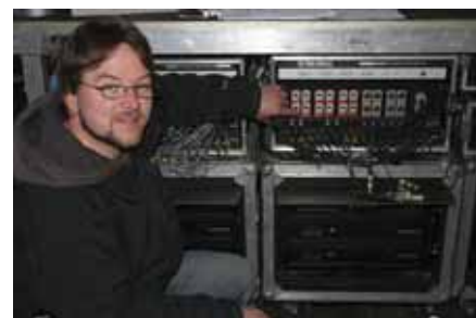
A team from TC Showtechnik led by Martin Schulze was responsible for both the planning and the implementation of the sound reinforcement design
