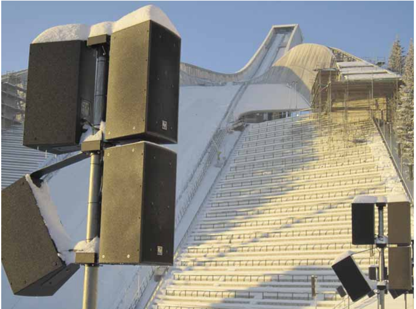
Electro-Voice loudspeakers provide sound reinforcement for the newly designed National Arena in Holmenkollen
